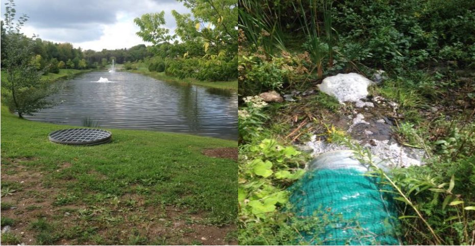
Figure 1D. Stormwater pond at Westview Village Retirement Home (left) and frothy, unsettled outflow (right) continuously releasing, slowly beginning to alter the natural forest vegetation towards a wetland complex.
